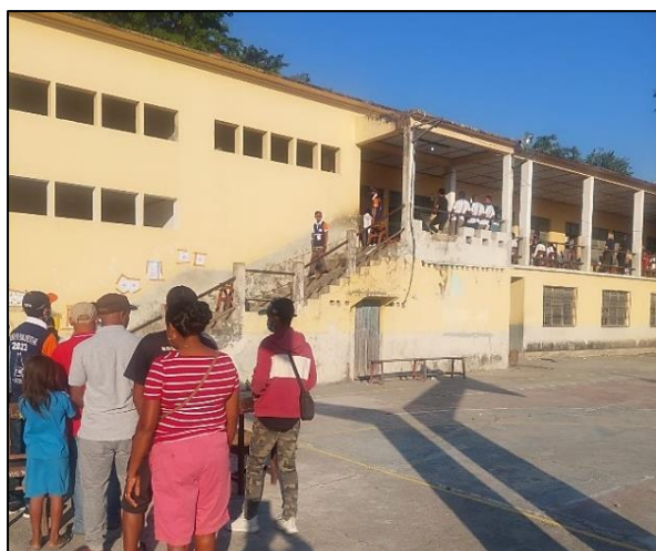
Photo 5: Stairs to access the station at Baucau villa Credit: Glenda Lasslett
